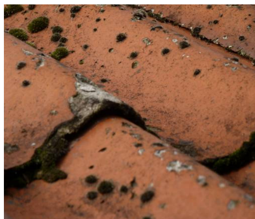
Friable roof surface (4.14)
